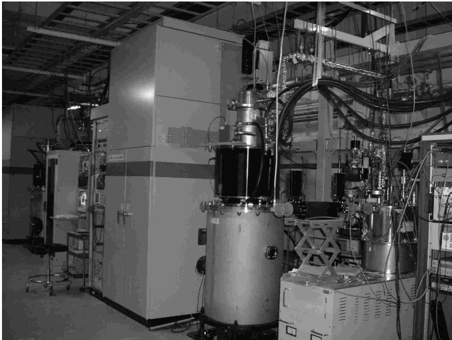
Figure 11.6: Klystron assembly and Modulator at KEKB linac 4-4 module
