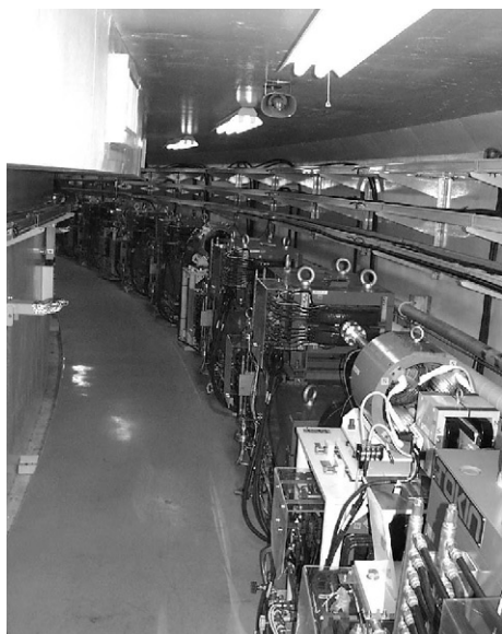
Fig. 3. Typical view from upstream at Arc-1.
